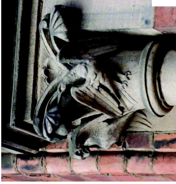
Wenlock Terrace – typical column head
